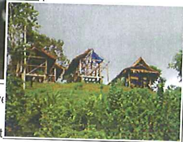
1st phase of leafhut construction
